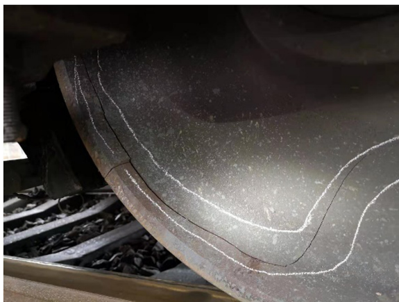
a circumferential crack of 468 mm
